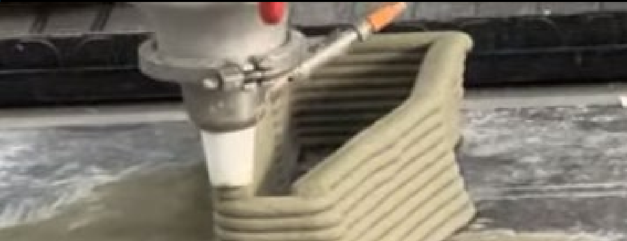
Close-up view of concrete additive 3d-printing, Vertico
